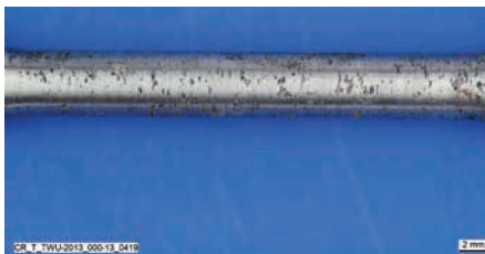
Stainless steel with pitting corrosion, e.g. A4 material used in a road tunnel
