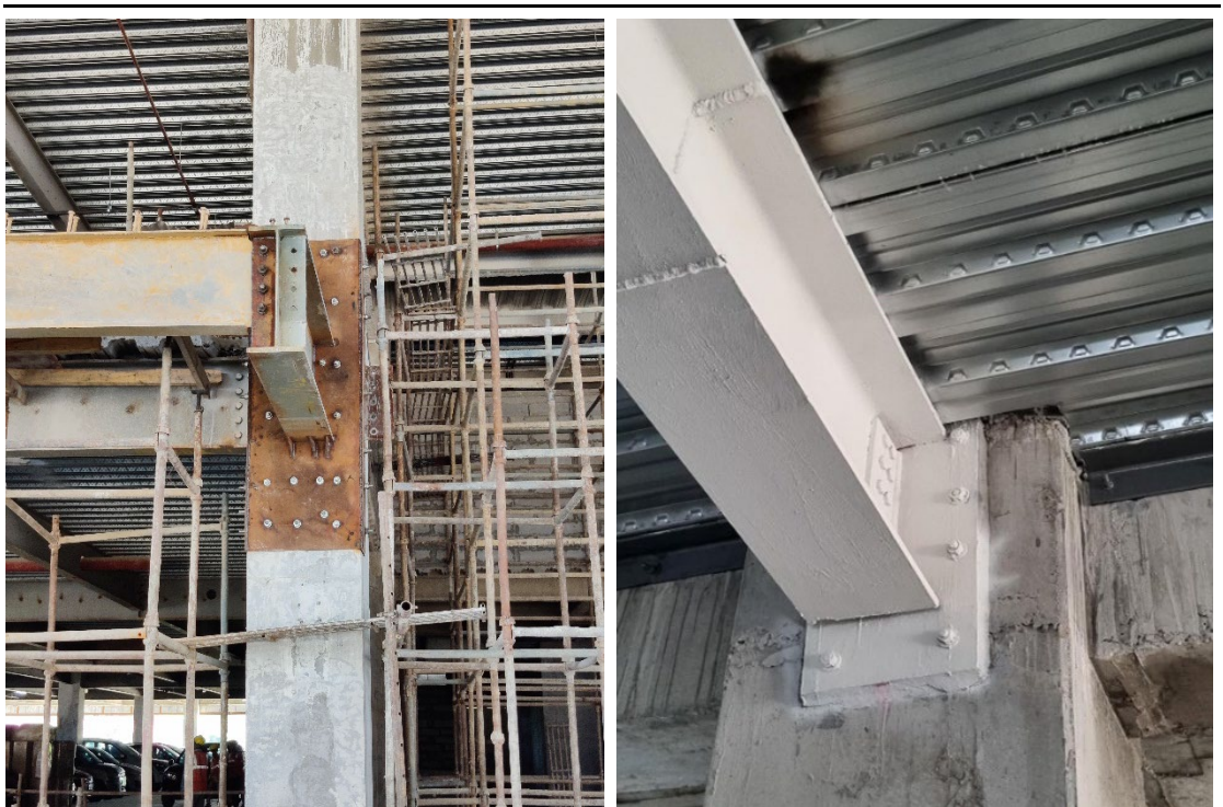
Fig. 1.1: Critical anchor arrangements at jobsite
