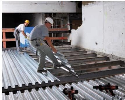
Figure 26: Installation phases for X-HVBs on profiled sheeting (from top left clockwise):
