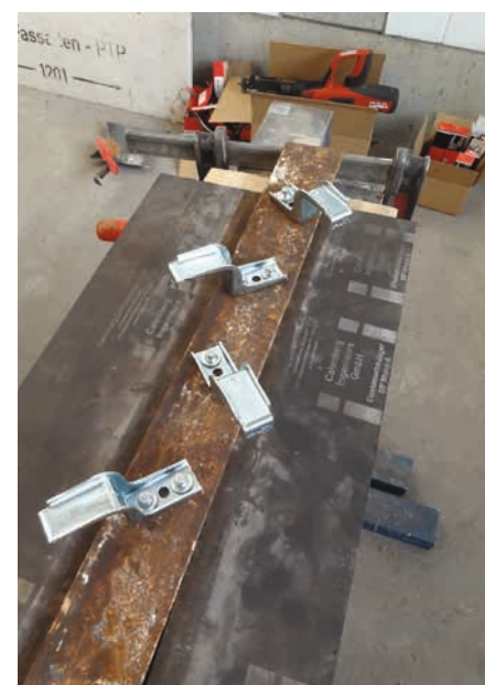
Figure 38: X-HVB installed with “duck walk” positioning on an old steel beam
