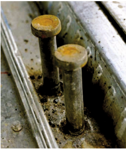
Figure 5: Shear studs welded on profiled deck
