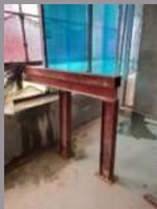
Heavy Duty Temporary Platform, Propping Crane, Support Passenger Hoist
